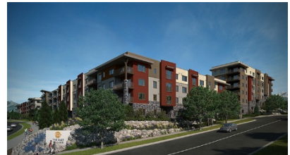
Sandy TOD – East Village Apartments
