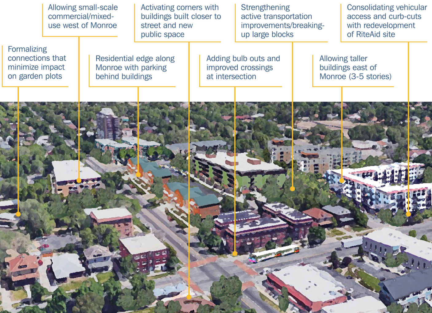
FIGURE 5.6 Key Elements of the 25th and Monroe Station Looking north from Monroe
