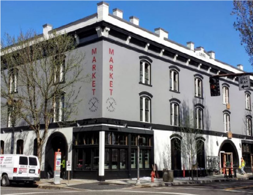
Enclosing the intersection and creating a gateway with taller buildings at the western side of the intersection
