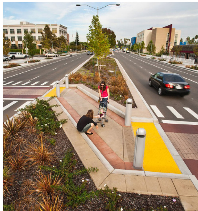
Providing well-defined and accessible crossings that provide visual contrast to pedestrians, cyclists, and motorists
